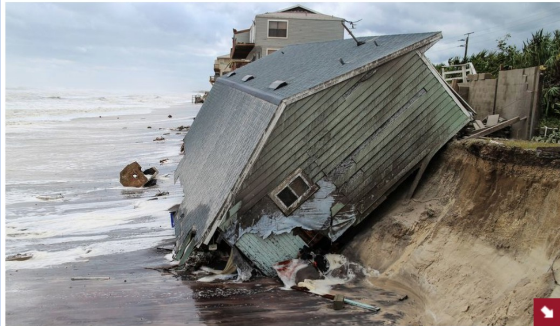
A house in Florida, slid into the Atlantic Ocean on Monday while Irma, downgraded to a tropical storm,
